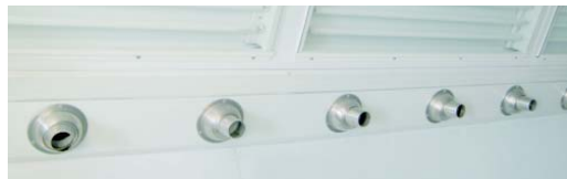
Water Painting Compliant
